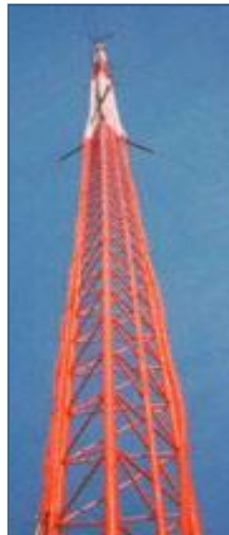
FCC-Compliant Paint Applied
