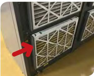
High-water mark on the filters and mud-slicked floor at KSBJ transmitter site.
