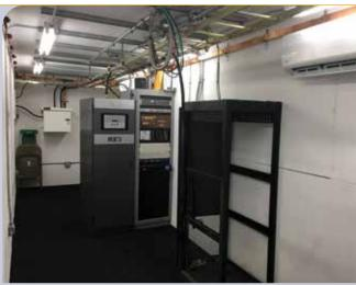
Inside the Lake Charles, LA, site. Two transmitters are yet to be moved in, one where the coax and wiring await. The other transmitter will be placed just out of frame. This installation occupies 28' of the 40' container.
